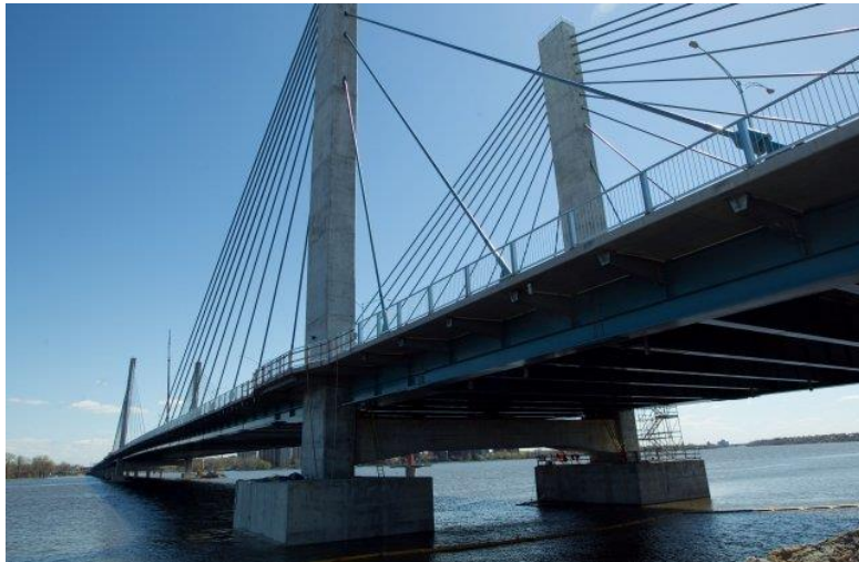
Completion of Highway 25 Laval-Montreal (Quebec)
